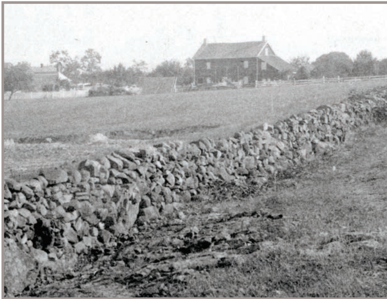
Stone wall along Brian Farm at Ziegler Farm, c1878. Upper right buildings are identified as the David Ziegler farm in this 1878 photo from NPS files.
