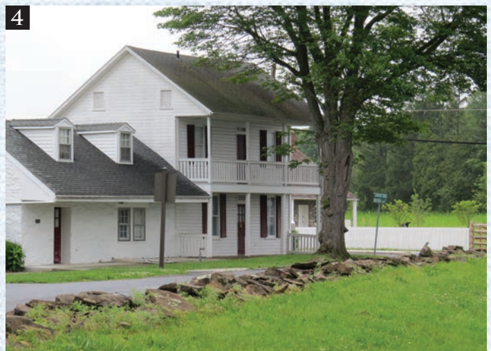
PHOTO 4: This is a part of a Confederate breastwork never used because it was constructed after the battle had ended. As Robert E. Lee started the long retreat back to Virginia, he wanted his Army of Northern Virginia wagon trains to be prepared in case of pursuit by Meade's Army of the Potomac on July 4 and afterward. Where is this line of defense and whose division was it?
