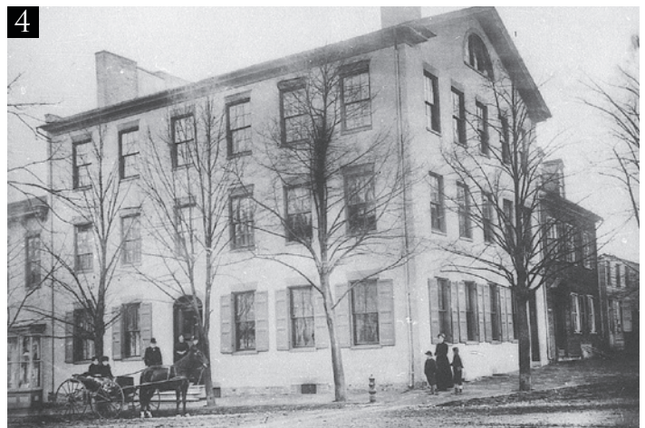
PHOTO 4: The structure in this photo holds a prominent place in the borough of Gettysburg today just as it did in the 1860s. It has been a family home, a law office, a drug store, an antique “mall.” It has been restored in part to its 1860s appearance and holds artifacts of the period and of the 16th President’s visit to Gettysburg, as well as offices on its upper floors. From a Tipton glass lantern slide.
