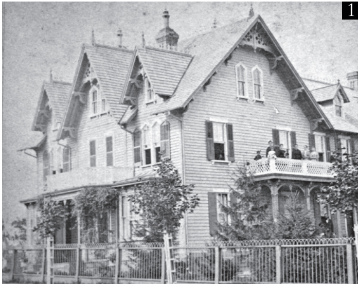
PHOTO 1: This house, sometimes called a “cottage home,” is no longer standing but its replacement, built in 1868, is on the original foundation. It was the site of fighting and army occupation during the Battle of Gettysburg. President Lincoln passed this house and neighboring houses on his way to dedicate a cemetery. Today it houses a small museum and offices. From a Tipton stereoview card.
